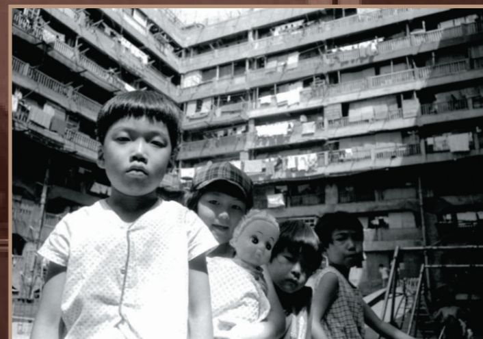
Children play in the shadow of one of the huge apartment blocks. (Right) The site as it looks today.
