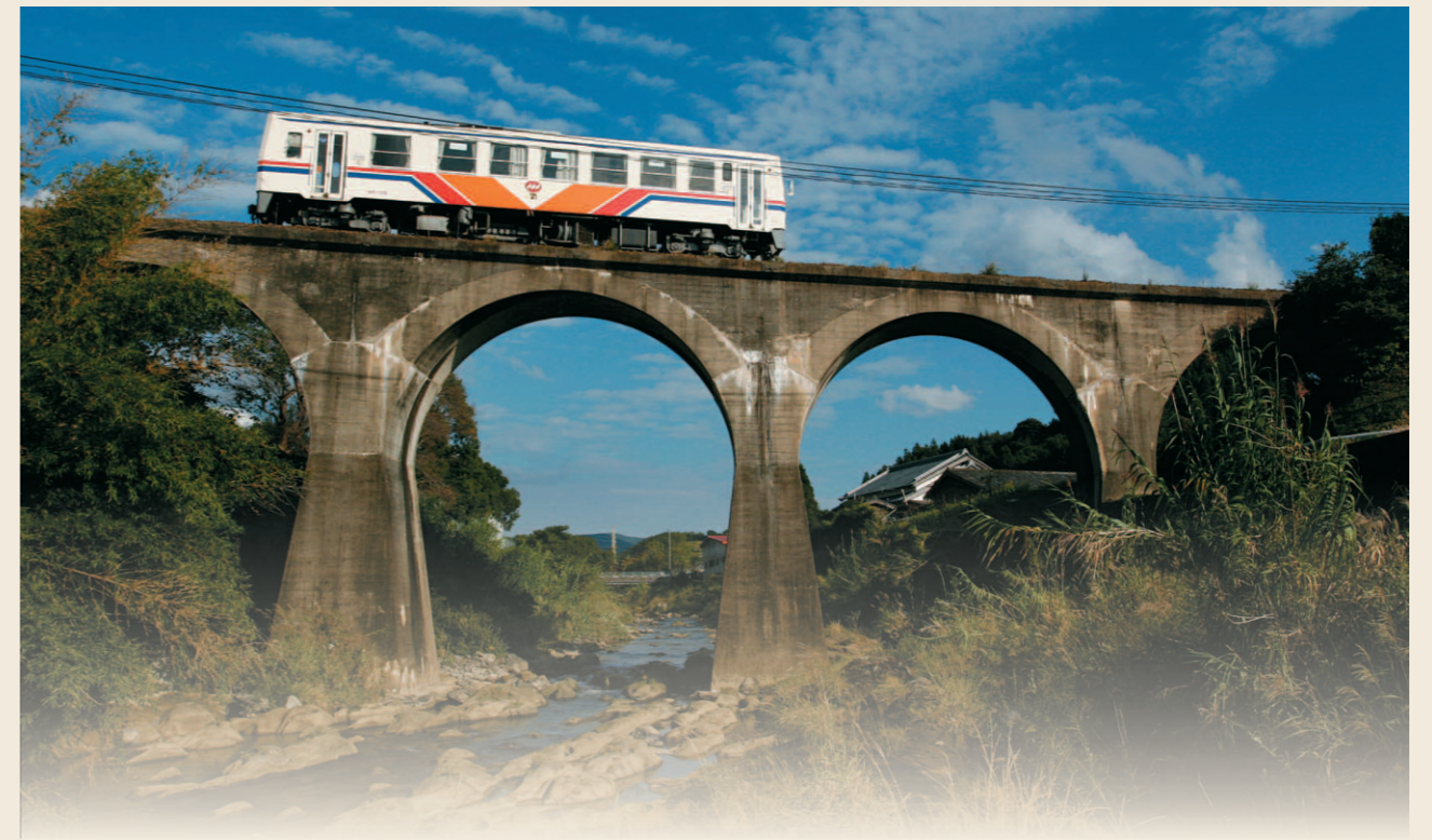
Yoshii River Bridge
