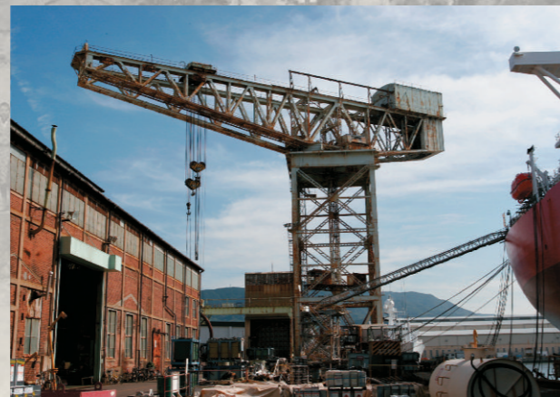
The 250-ton cantilever crane built by Sir William Arrol & Co. of Glasgow in 1913 is still operating today in the Sasebo shipyards. Of three cantilever cranes remaining today in Japan, two are located in Nagasaki Prefecture.
