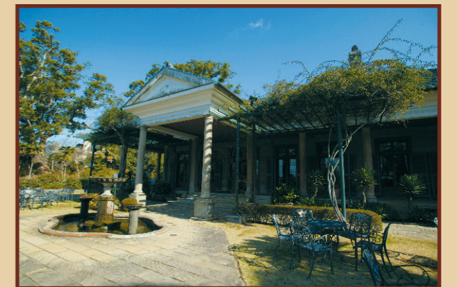
Erected in 1865, the former Alt House evokes an elegant fusion of Japanese and European architectural styles, including what is probably the first European fountain built in Japan.
