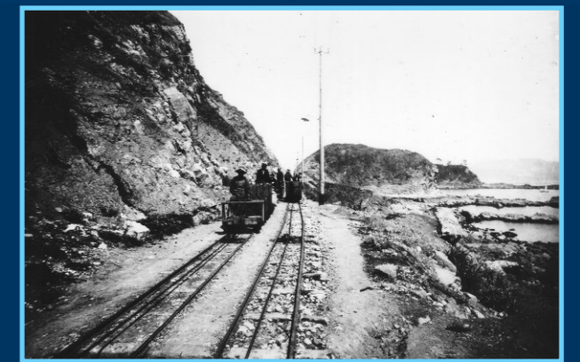
Thomas Glover laid tracks along the coast of Takashima Island to transport coal.
