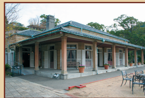
Like the former Glover and Alt houses, the former Ringer house is a national important cultural asset and a rare example of architectural collaboration.
