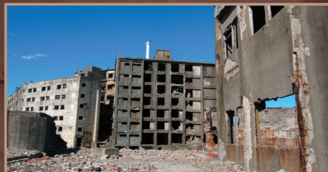
Erected in 1916, building No.30 (center) was the first large-scale reinforced concrete building in Japan.
