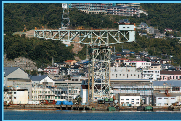
The Scottish-built cantilever crane has a height of 61 meters tall, an arm reach of 73 meters and a lifting capacity of 150 tons. It is still in operation more than a century since its installation.
