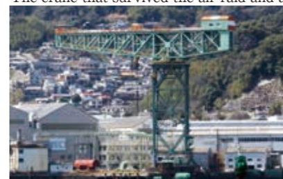
Mitsubishi Heavy Industries Ltd.
