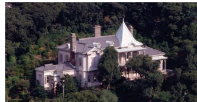
Mitsubishi Heavy Industries Ltd.
