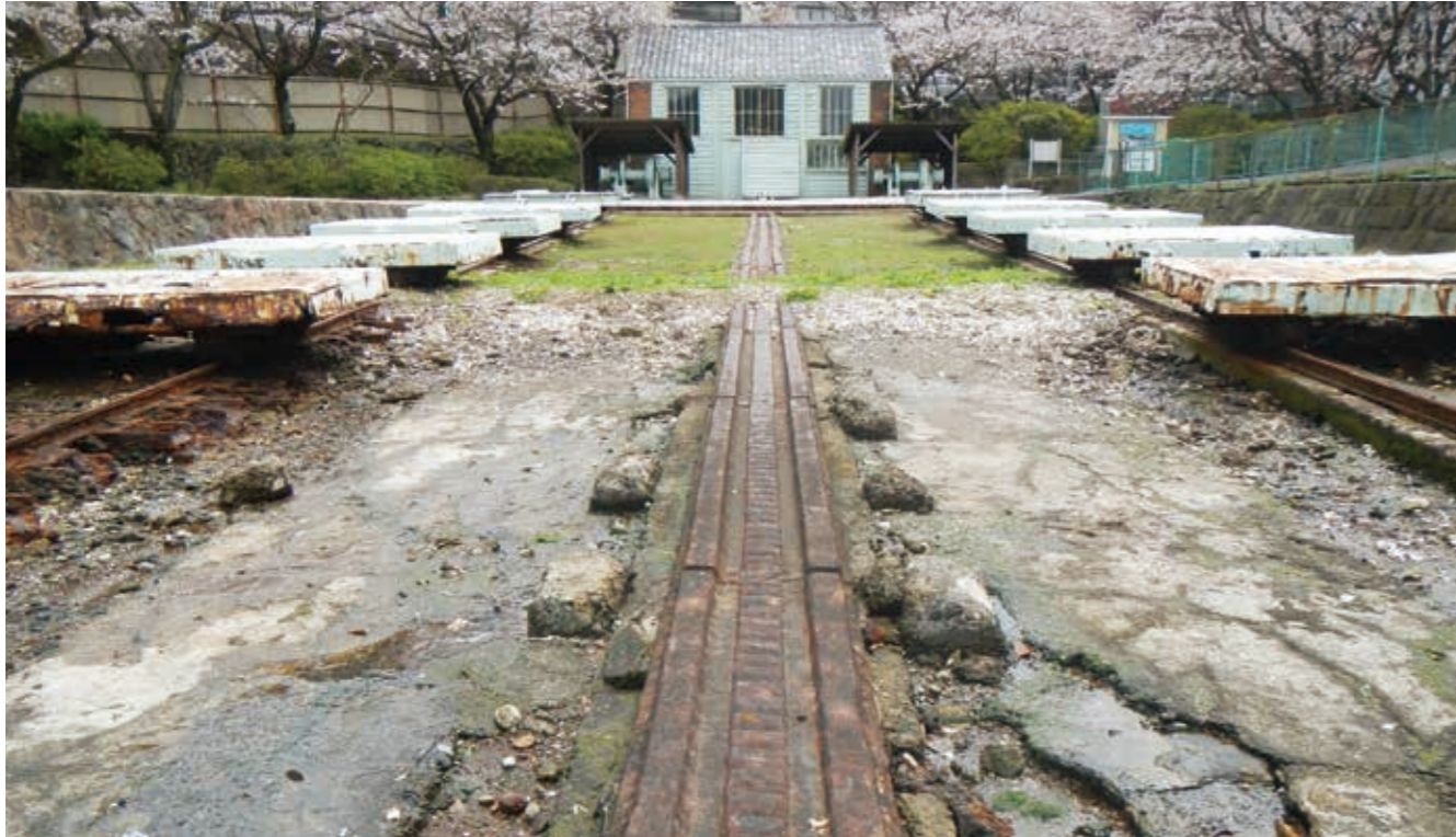
Mitsubishi Heavy Industries Ltd.
