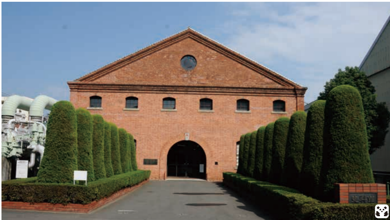
Mitsubishi Heavy Industries Ltd.
